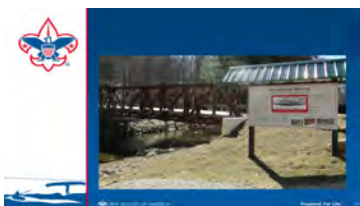
Sign and bridge (A)
